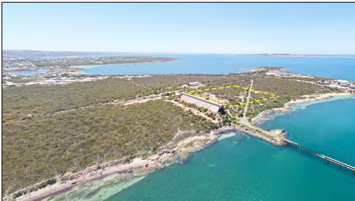
Figure 3 - View showing proposed Desalination Plant footprint (in yellow) adjacent to disused BHP infrastructure. The Historic Jetty is shown in the front right of frame (image courtesy of Applicant)
