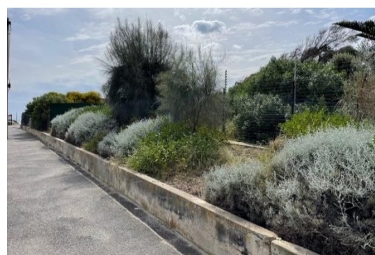
Local species planted in high densities to produce a novel and structurally diverse ecosystem, which fulfils multiple services at SA Water's Glenelg Wastewater Treatment Plant. Photo: G Garrard
