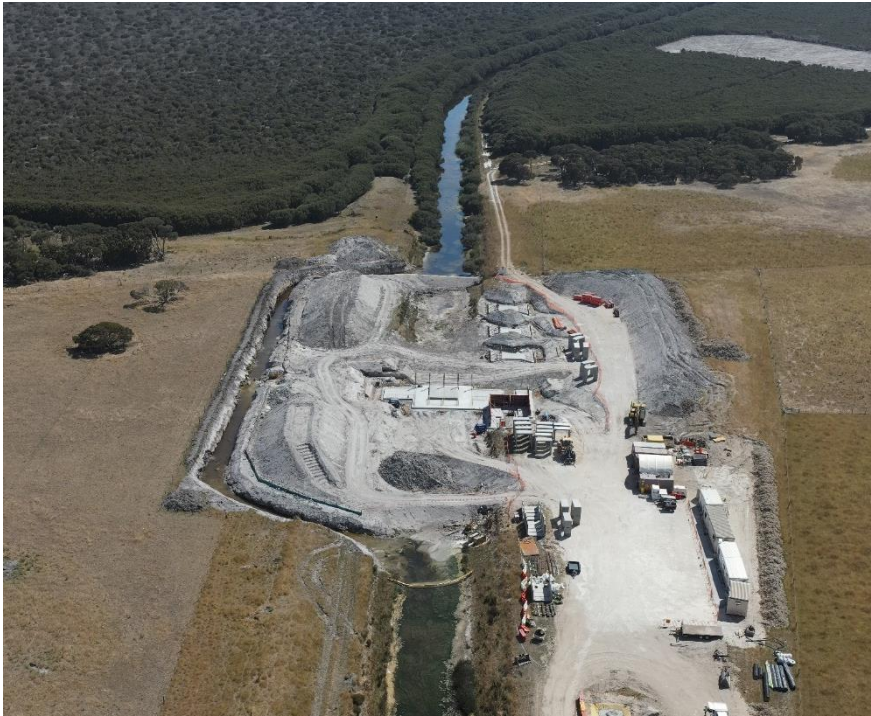
Lake Hawdon North weir Project 2024
