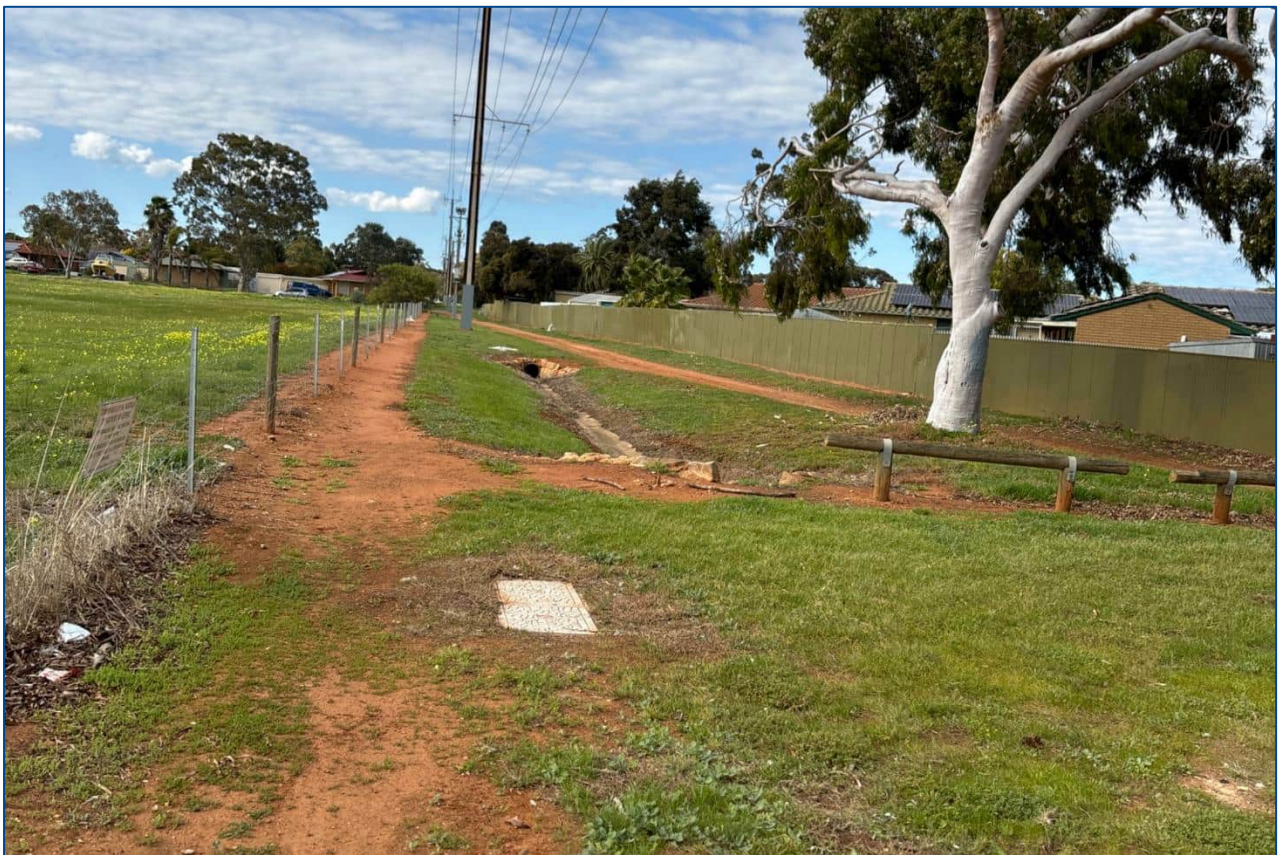
Figure 8: Property's south offsite drainage
