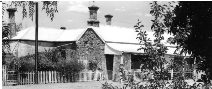
(SH-10066) 1979, House (former Devonshire Hotel)
