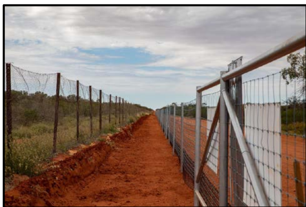
Example of similar fence construction (on right) along the SA/NSW border at the Hungerford pilot site (image courtesy of the Applicant)
