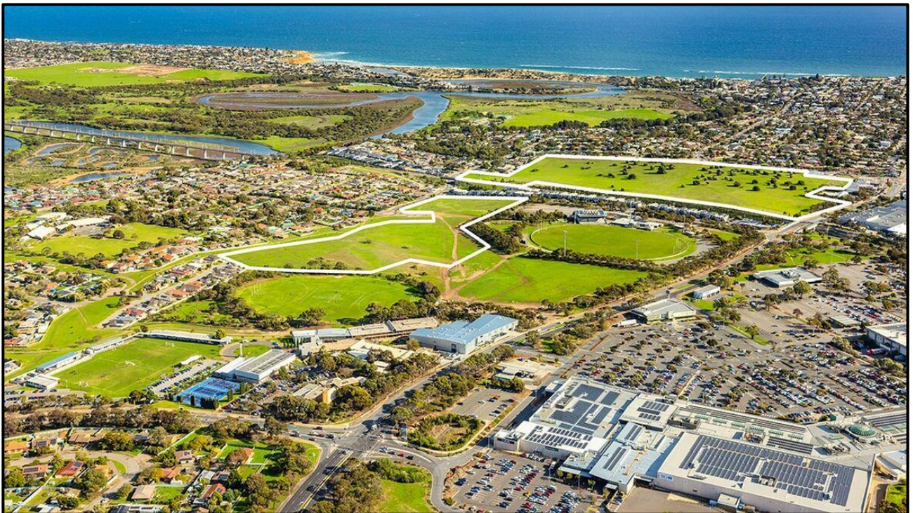
Figure 1 – View of parts of the Application Areas indicatively outlined in white looking south-west (image courtesy of the Applicant)
