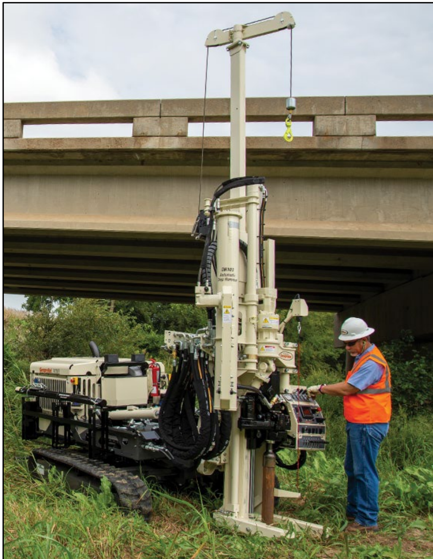
Figure 3 – Image of a drill rig in use (courtesy of the Applicant)
