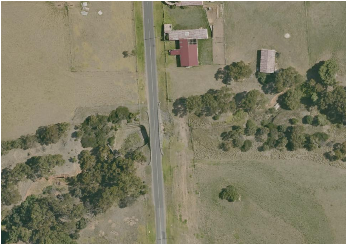
Figure 2.9 Existing bridge on Country Road across Sellicks Creek (source: Location SA MapViewer)
