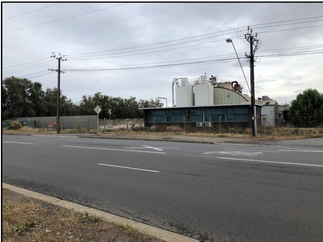
Figure 1 – Eastern Parade, Gillman facing north-east (image courtesy of the Applicant)
