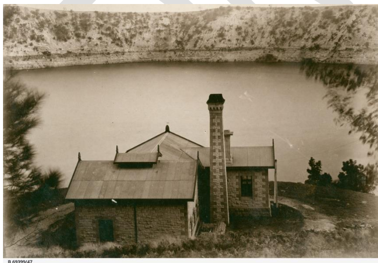
Blue Lake Pumping Station, circa 1920. State Library of South Australia, SLSA B 69399/47
