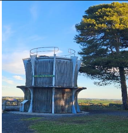
Keegan Drive surge tank DEW 2024
