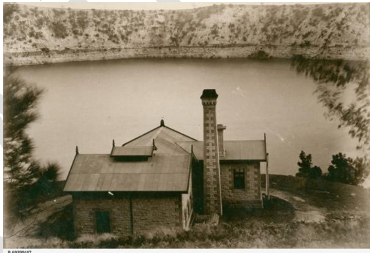
Blue Lake Pumping Station, circa 1920. State Library of South Australia, SLSA B 69399/47
