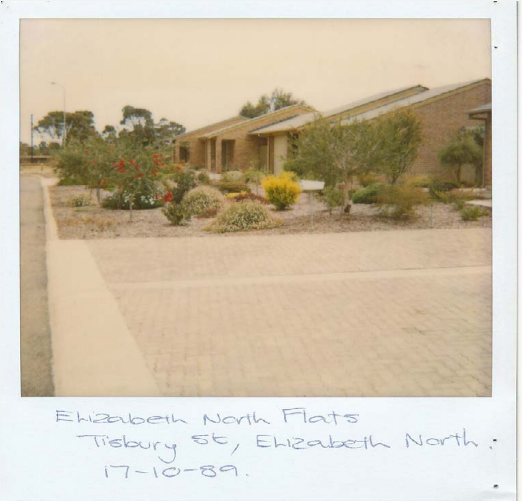
Semi-detached housing delivered by the SA Housing Trust in the 1980s
