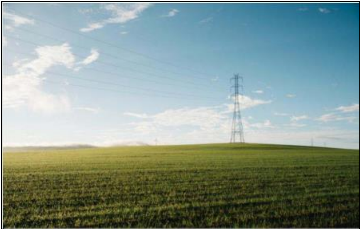
Figure 4 - Typical example of transmission lines and towers (image courtesy of the Applicant)
