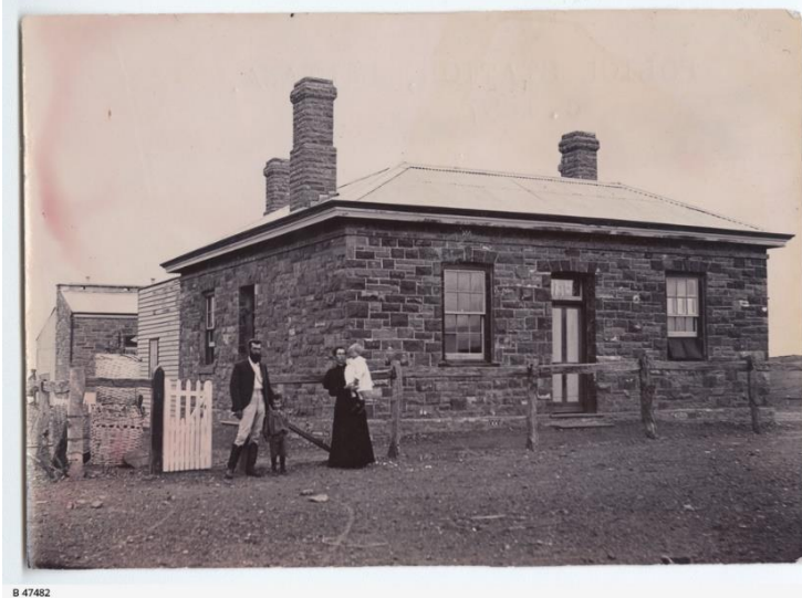
Police Station, Beltana, 1897, State Library of South Australia, SLSA B-47482
