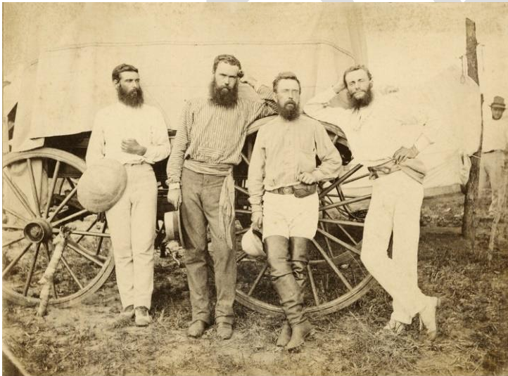
Overland Telegraph Construction Party, John Little, A. G. Patterson, Charles Todd and A. J. Mitchell, 1872, State Library of South Australia, SLSA B-4639
