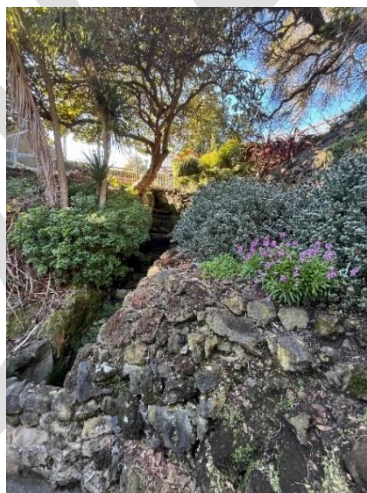
Rock faced walls of Mount Gambier limestone rubble reflects the Gardenesque style, and adds a naturalistic feature to the garden's design, DEW 2024
