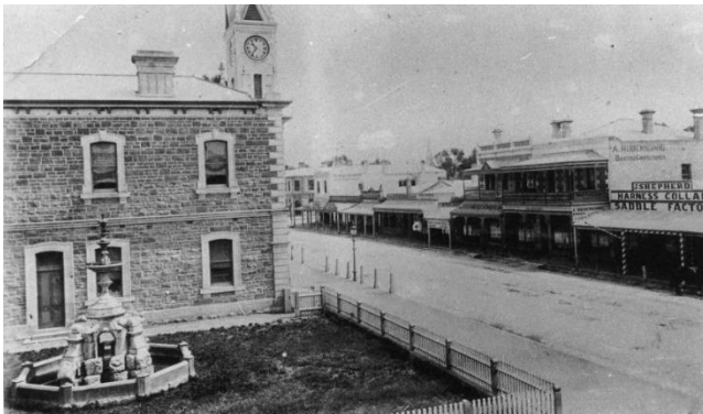
View of the old Town Hall in 1895, looking north-west, showing the Gardiner Fountain, with the former Jens Annexe / Rubenkonigs Coffee Palace opposite, Les Hill Photographic Collection, Mount Gambier Library, MT 24F19 D00011977
