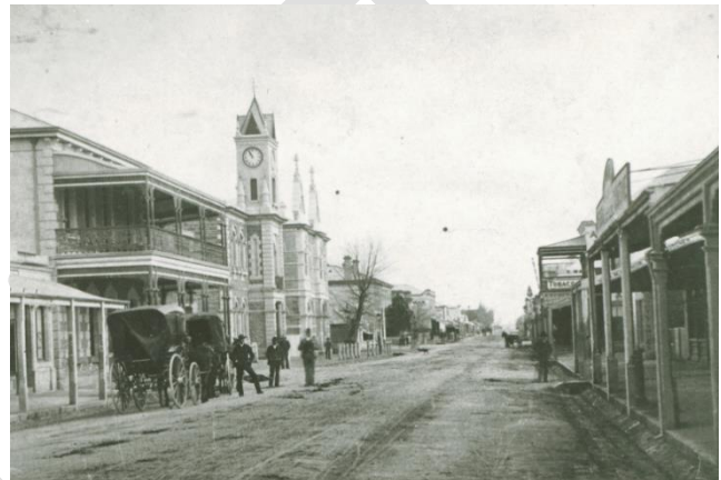
View of Commercial Street, looking west, showing the corner of Jens Hotel on the left with the old Town Hall and Institute buildings beyond, c.1890, State Library of South Australia, B13430
