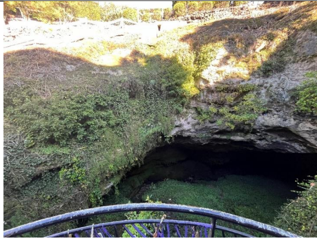
View into the sinkhole from viewing platform within the Cave Garden, DEW 2024
