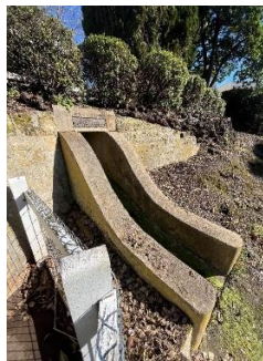
The stormwater channel, constructed 1916 under the supervision of engineer F. N. Burchell, manages rainfall and urban runoff flows on the steeply sloping banks of the sinkhole; in rainy weather, a waterfall is formed, DEW 2024
