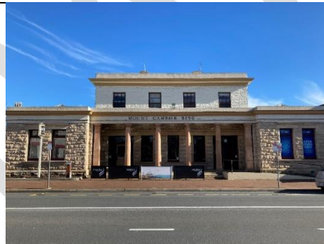
Mount Gambier Post Office (Former Telegraph Office), DEW 2024
