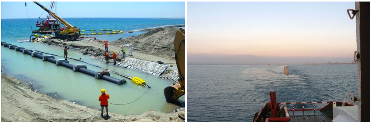
Desalination plant intake and outfall pipelines using float and sink methodology
