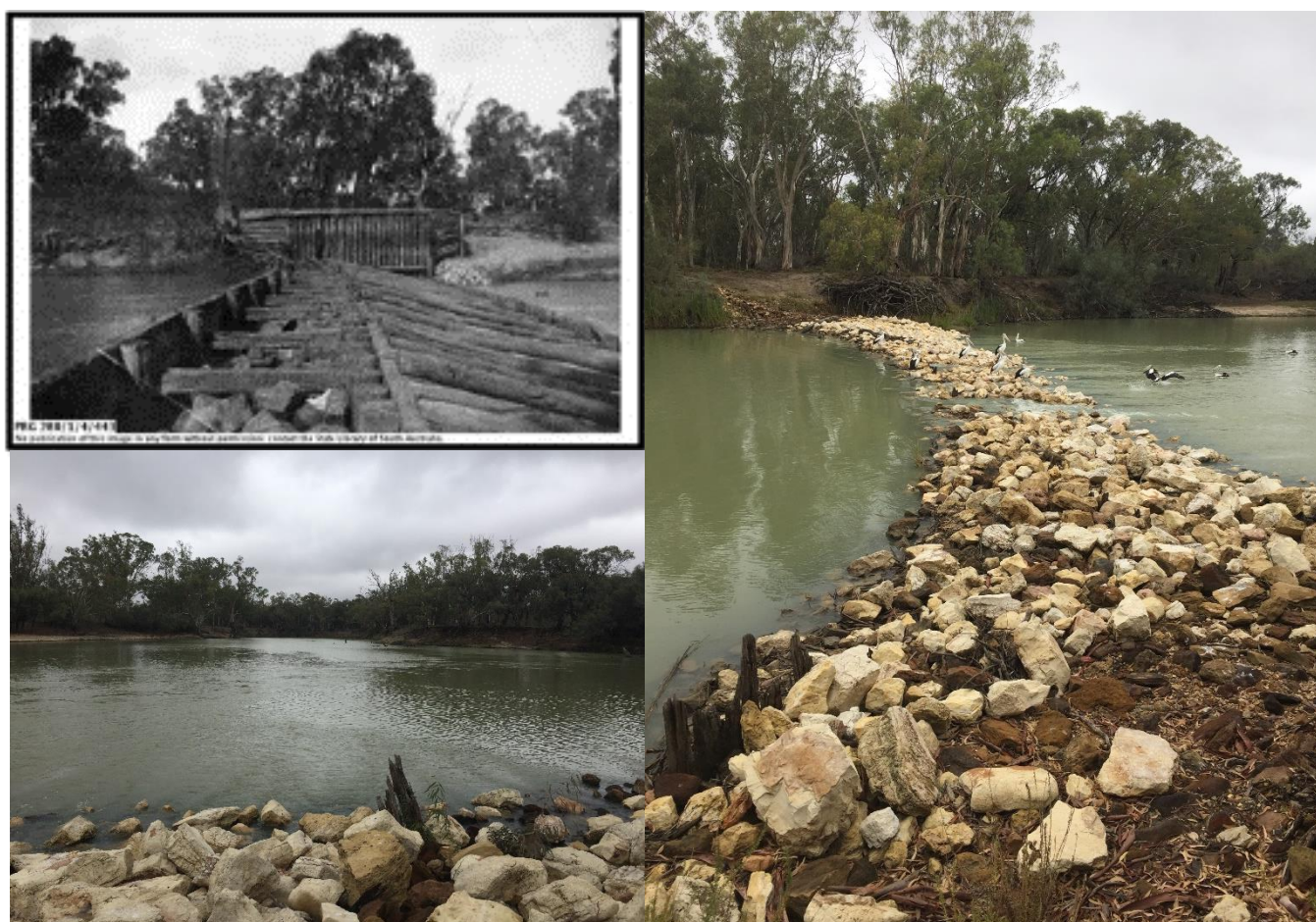
Pictures: Top left, historic picture of the stone-filled timber crib weir; Right, current condition of Stone Weir (March 2020); Bottom left, on top of Stone Weir, looking downstream (March 2020).
