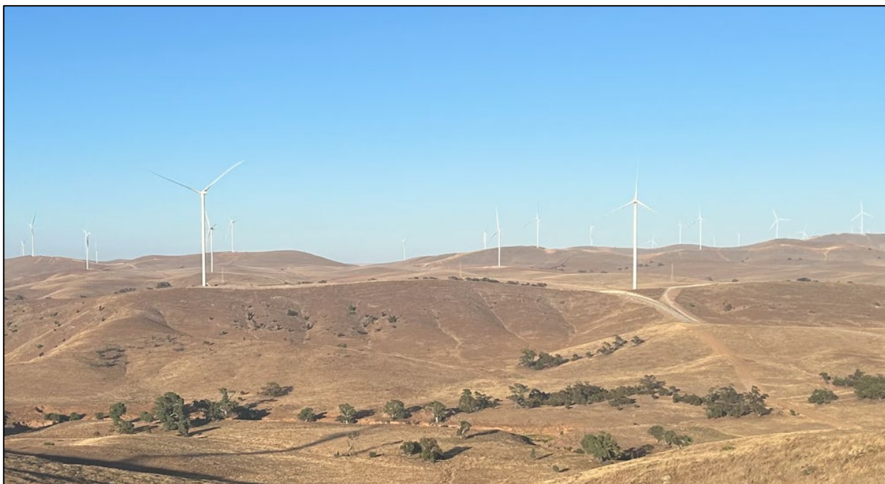
Figure 2 - Wind turbines in the Goyder South Hybrid Renewables Energy Project area (courtesy of the Applicant)
