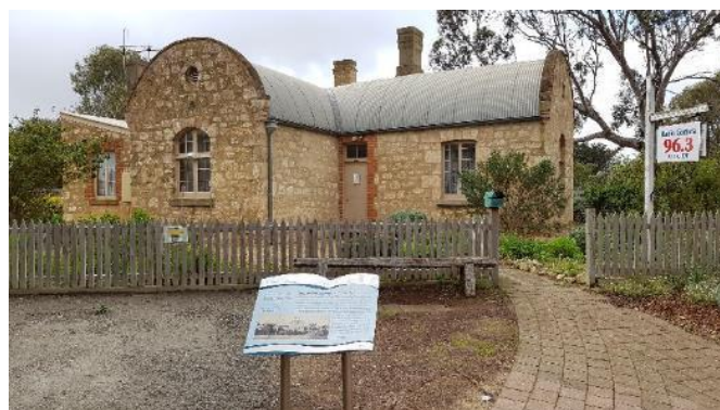
Railway Superintendent's House (State Heritage Place No. 10469) commenced 1852, showing the typical materials palette of limestone masonry with face brick quoins and stone and brick window surrounds. DEW 2016
