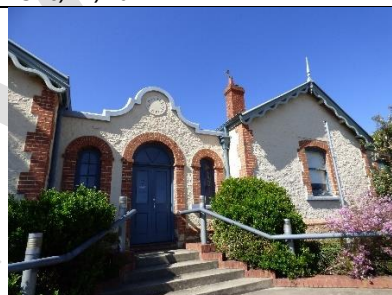
View of the entrance to the Goolwa Police Station and Courthouse (SHP 10368), begun in 1859 and completed in 1867, showing vertically-proportioned, timber-framed, sash windows with brick quoins. DEW 2019
