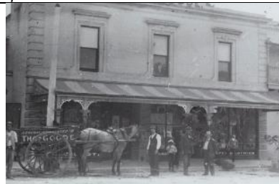
Thos. Goode's Store, Cadell Street, showing corrugated iron verandah, then painted with Federation-style contrasting stripes. Photo: c.1915 (Courtesy of State Library of SA)
