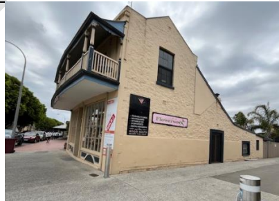
Bow-Fronted Shop, Cadell Street, c.1850s (State Heritage Place No. 10358). The front wall of the store follows the allotment boundary, giving a bow-shaped appearance. Note the steeply-pitched lean-to. DEW 2024
