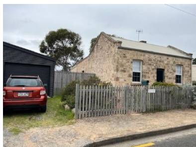
View showing two successive lean-to additions built to the rear of a cottage in "Little Scotland". DEW 2024
