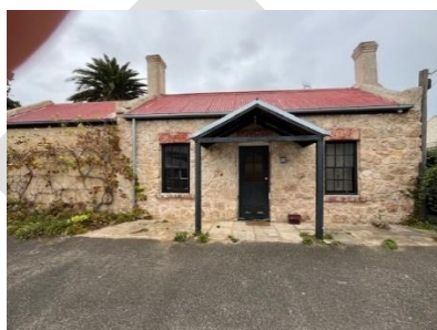
Typical masonry cottage in the "Little Scotland" precinct. The portico is a later addition. DEW 2024
