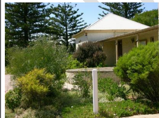
View of Customs House towards Cutting Road, with its replanted landscaping and avenue of Norfolk Island pines (DEW).
