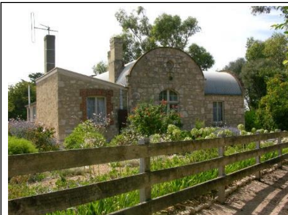
View of the Railway Superintendent's House, with cottage garden plantings contrasting with remnant native vegetation including eucalypts and ti-tree (DEW 2005).
