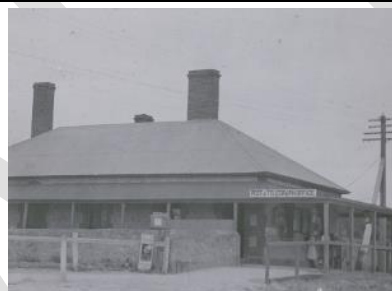
Goolwa Post Office (1857, with later additions), showing the simple pitched roof form. State Library of South Australia, c.1920, PRG 1316/12/204
