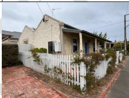
Typical low, open fencing in the "Little Scotland" precinct. DEW 2024
