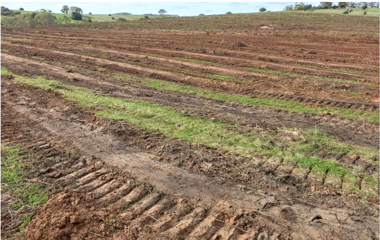
Figure 7: Typical Site Condition (Facing South-East)
